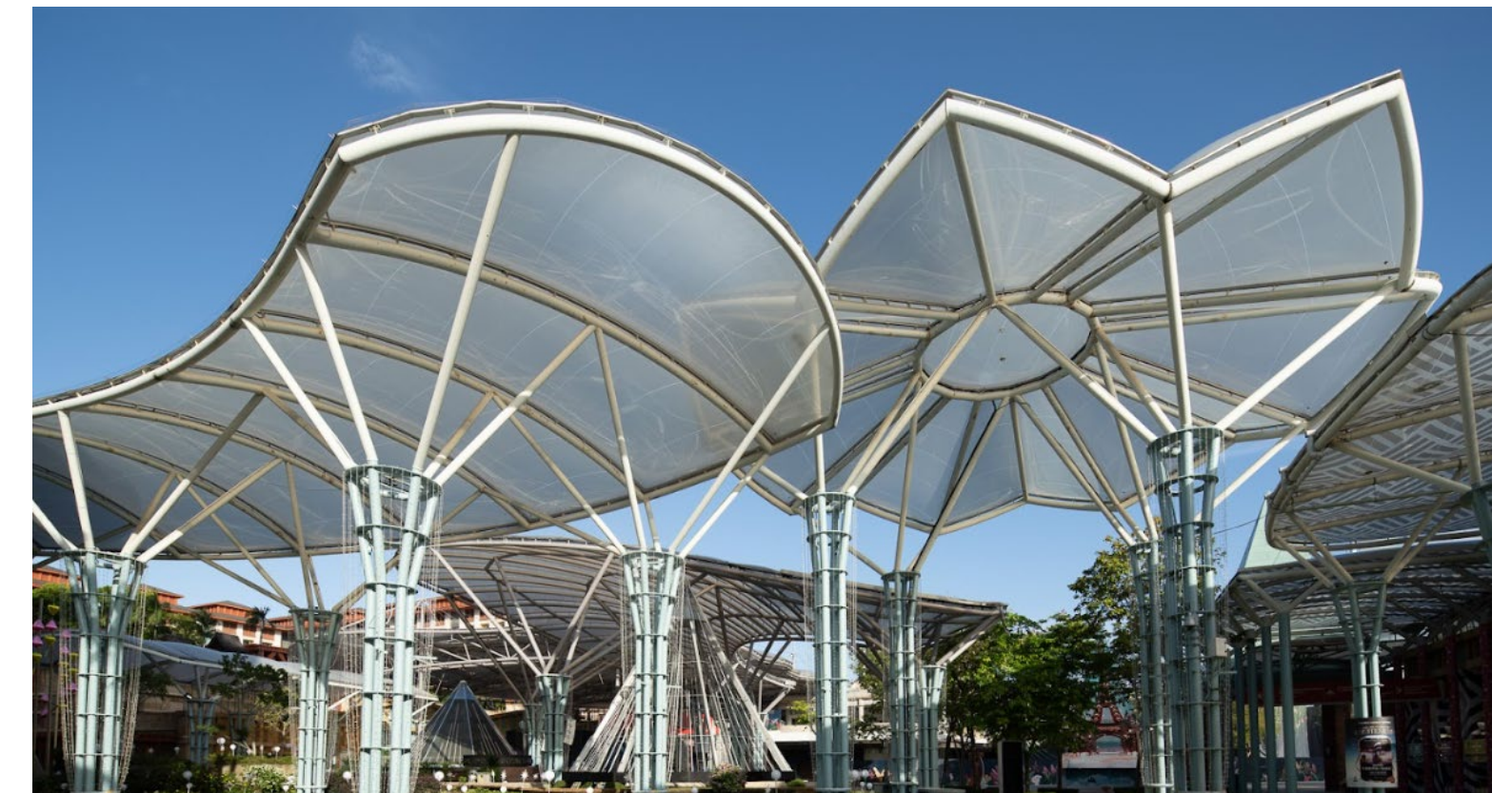
ETFE roofs installed across RWS to improve thermal comfort
