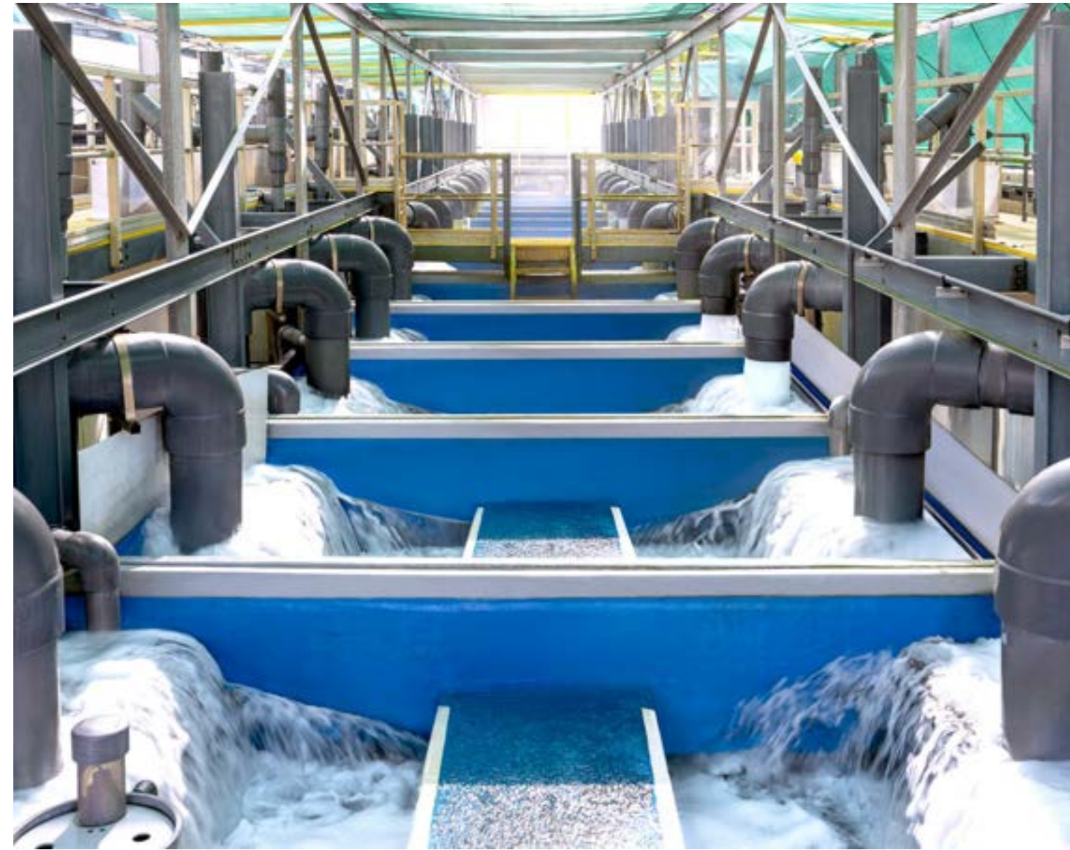
View from atop our foam fractionators cleaning and filtering seawater used for S.E.A. Aquarium
