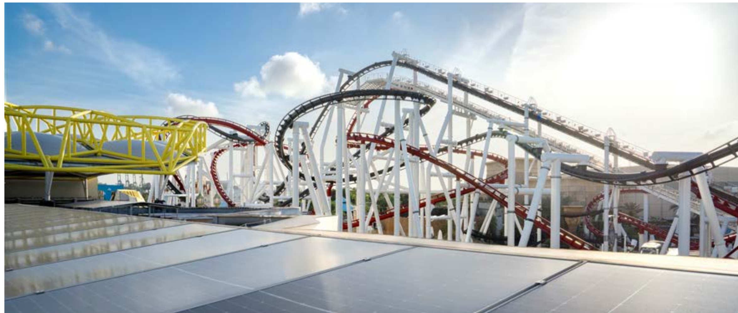
Universal Studios Singapore rooftop solar panels
